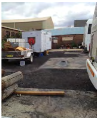
View of the burnt down building footprint Looking north
